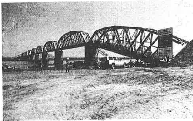
Railroad Bridge in Mozambique That Was Repaired With Child Survival Funding Photo: USAID
